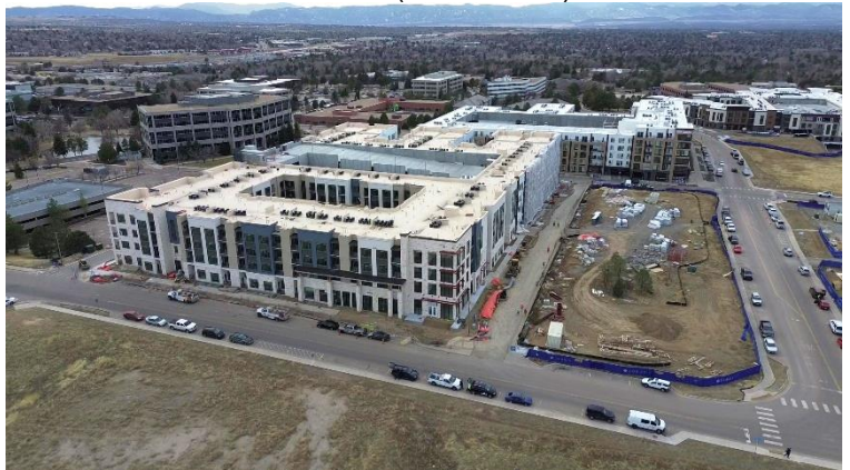
Parcels 6 & 7 (View: Southwest)
