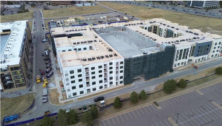
Parcels 6 & 7 (View: Northeast)
